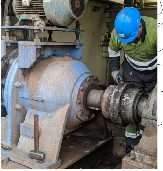
Disconnect the coupling that connects the screw shaft to the gearbox stub shaft.
