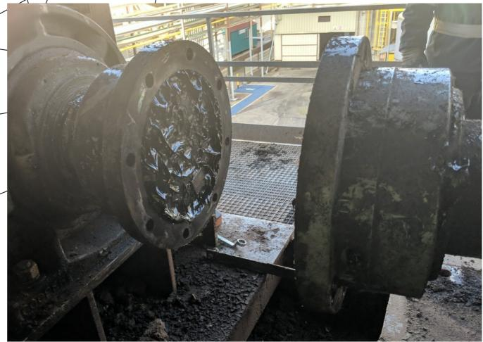
Move the gearbox and motor out of the way.
