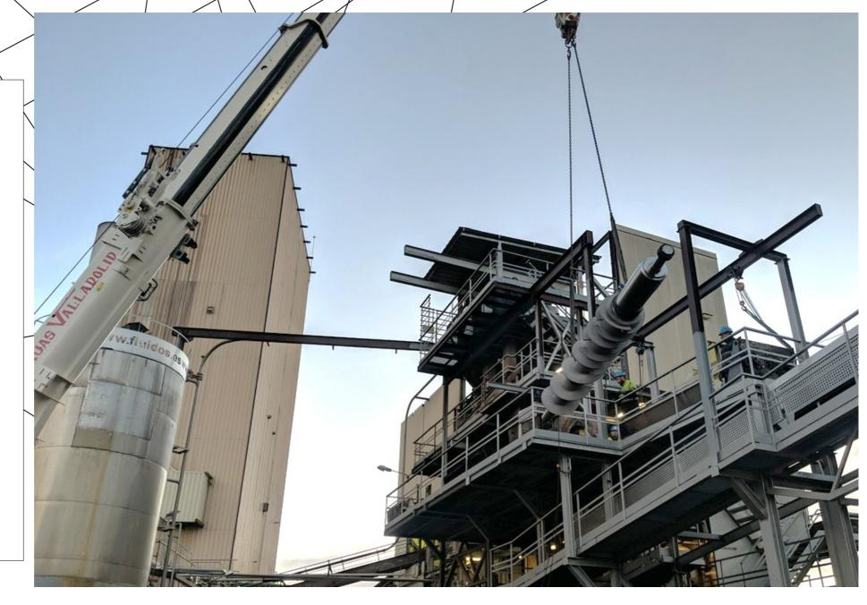
With the new screw in place, the coupling hub is heated and installed.
