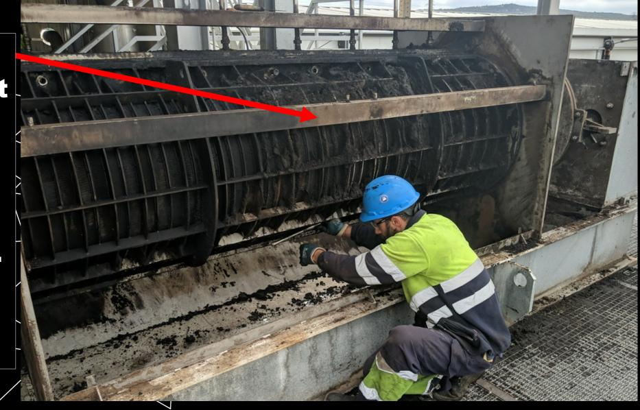
**The Resistor Bars** are sandwiched between the two screen halves. After removing the screens, remove these **Resistor Bars.**
